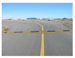
A single solid yellow line and a single dashed yellow line mark the boundary between the *Non-movement Area* (the area NOT controlled by ATC) and the *Movement Area* (the area that is controlled by ATC).
